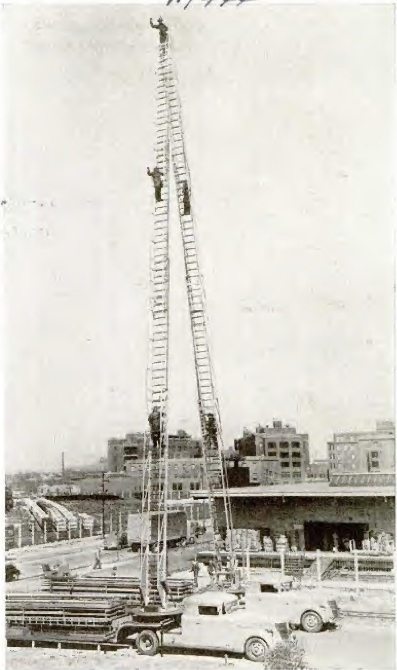
Huge steel ladders, hydraulically operated, make portable fire escapes
